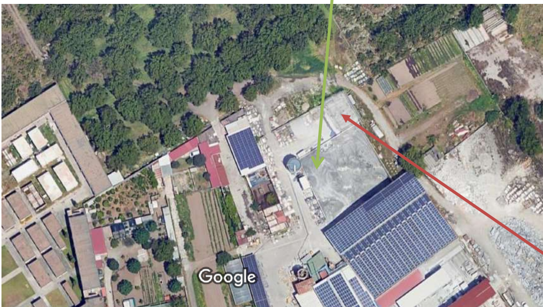
SLUDGE STORING POOL
